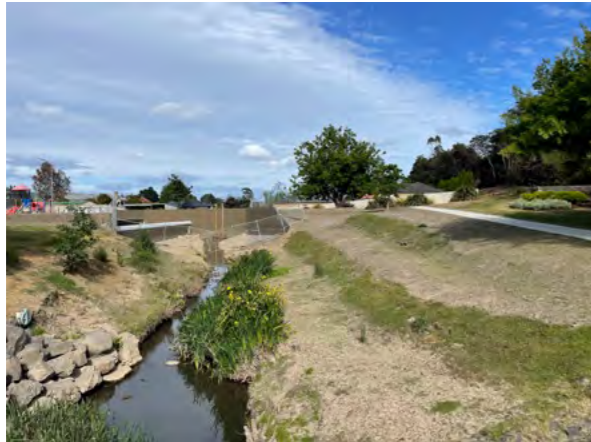
Existing flood levy in Kings Park
