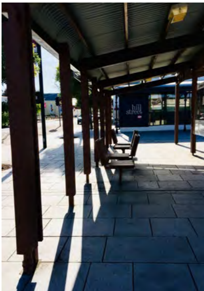
Existing canopy structure in the plaza
