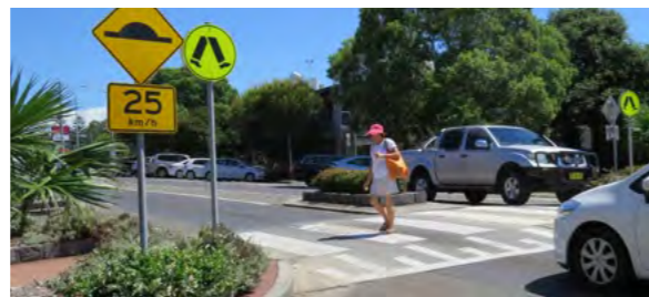
Examples of raised pedestrian crossing
