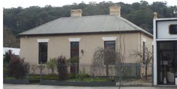
Good example of fencing outside 133 Gilbert St
