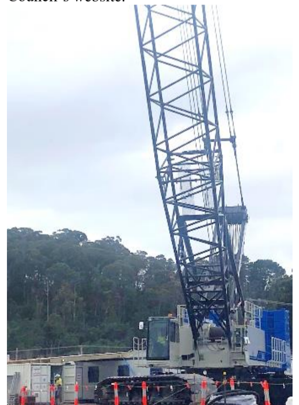
Image: 275-ton crawler crane
