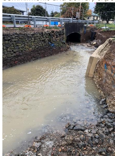
Bonneys Creek Culvert
