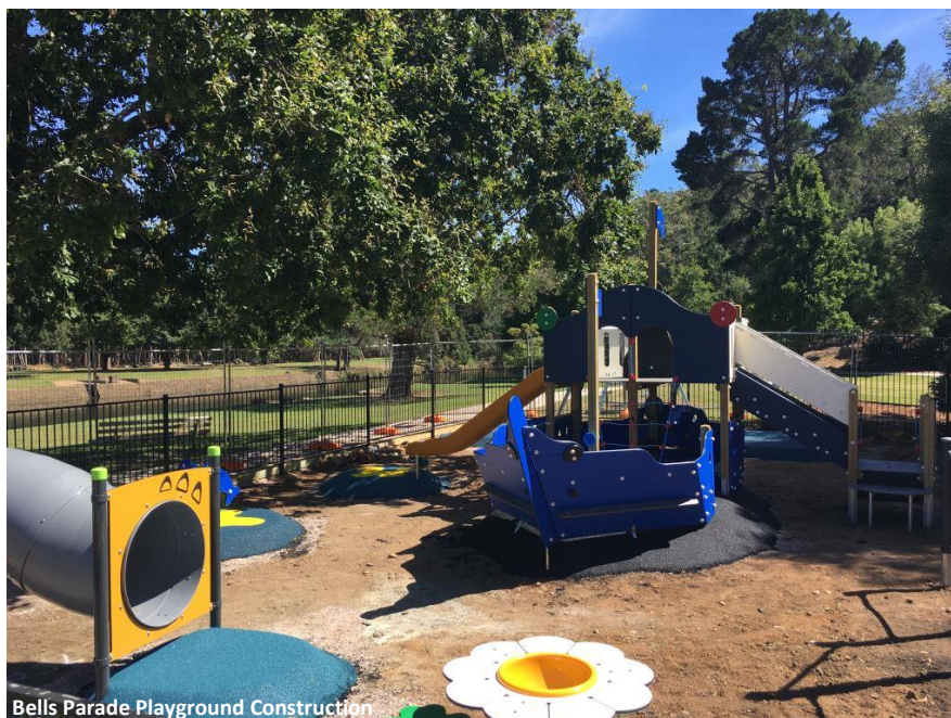
Bells Parade Playground Construction
