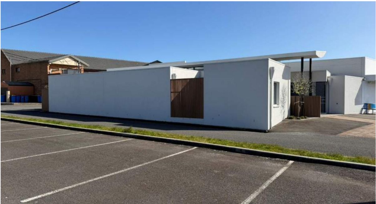
Figure 5 22 Shearwater Blvd, view from carpark to the south.
