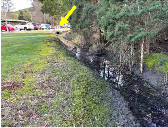
Drain looking south-eastwards towards terminal culvert/pipe (arrow)
