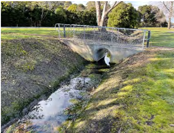
Walking track over bridge across drain
