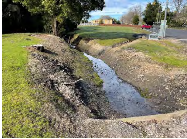
Terminal drain culvert/pipe looking south-eastwards
