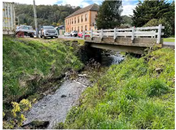
Kings Creek passing under bridge on Victor Street
