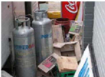
Not clear from combustibles or secure
