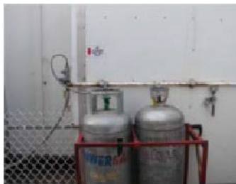
Secured and clear of combustibles
