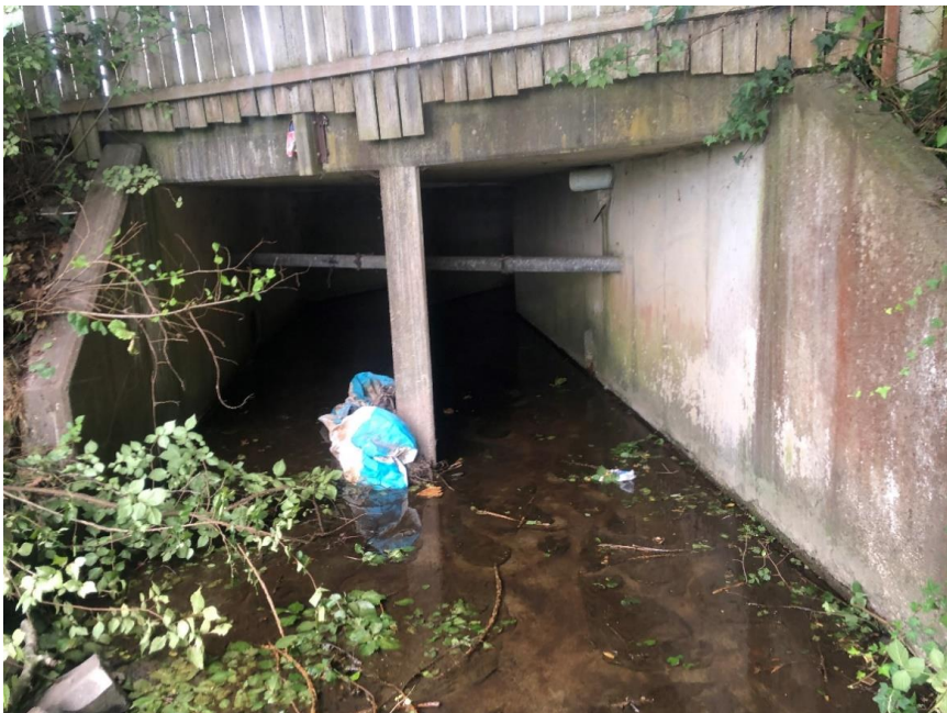
Figure 2.4: Moriarty Road crossing (looking downstream)
