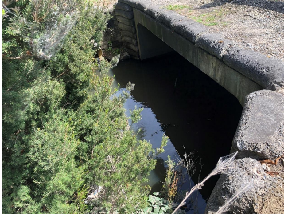
Figure 2.5: Percival Street crossing (looking downstream)
