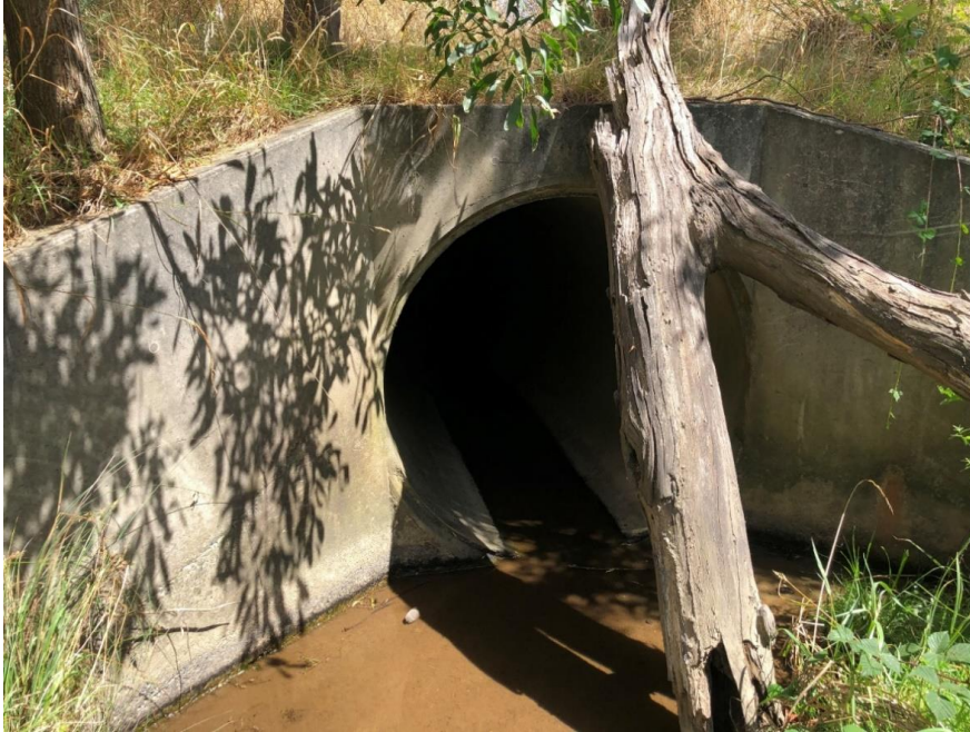
Figure 2.3: Outlet pipe under Bass Highway
